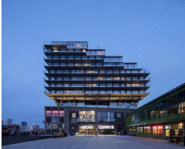
Gambar 2.48 Fenix I Warehouse Renovation
