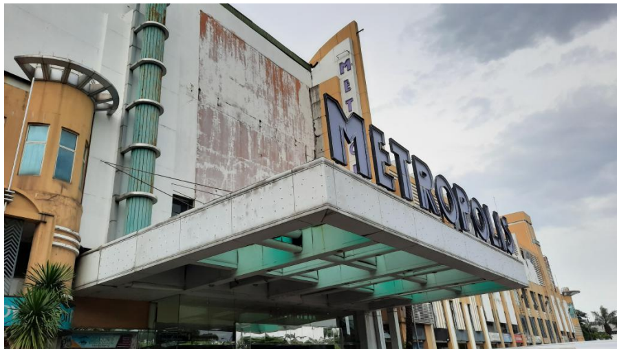
Gambar 1.4 Kondisi bangunan Metropolis Town Square
