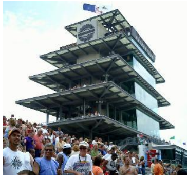
Gambar 2. 8 Race Control Tower
