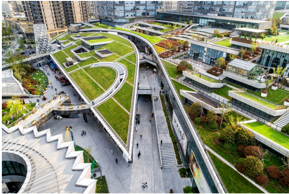
Gambar 2. 11 Green Roof Shanghai Greenland Centre
