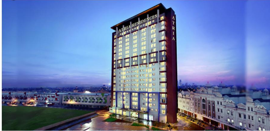
Gambar 2.4 Gedung Atria Residences
