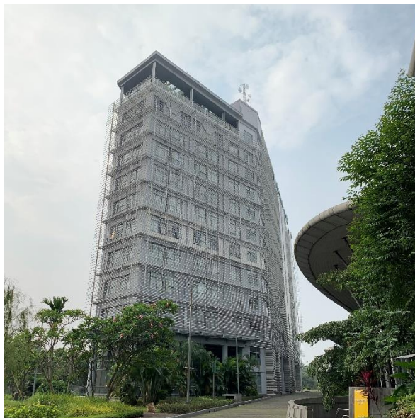
Gambar 2. 2 Gedung Hotel Santika Premiere ICE - BSD City
