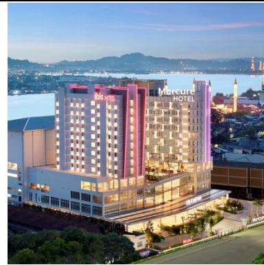
Figure 2.3 Mercure Hotel Samarinda' Building
