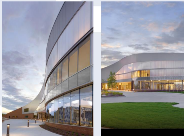
Gambar 2. 9 Maryland Heights Community Recreation Center
