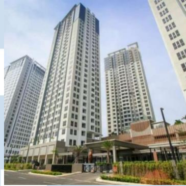
Picture 3.1 M-Town Residence
