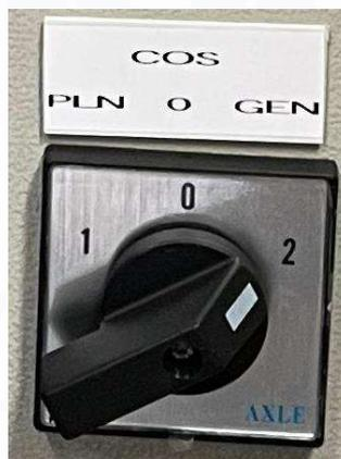
Gambar 3.8 *Selector Switch AXLE 1-0-2*
