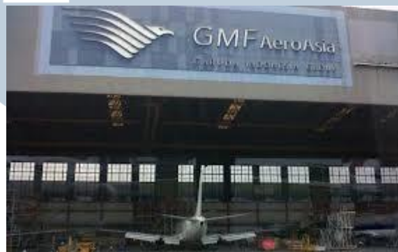
Gambar 2.4 Hanggar PT Garuda Maintenance Facility Aero Wisata
