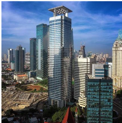
Gambar 1.1 Gedung Sinarmas MSIG Tower
