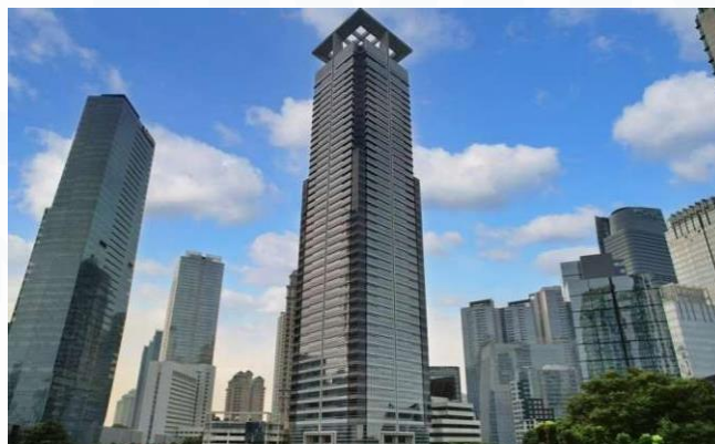
Gambar 1.1 Gedung Sinarmas MSIG Tower
