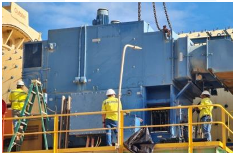
Figure 1. 2 Motor 6750 kW 11 kV for Mining Industry
