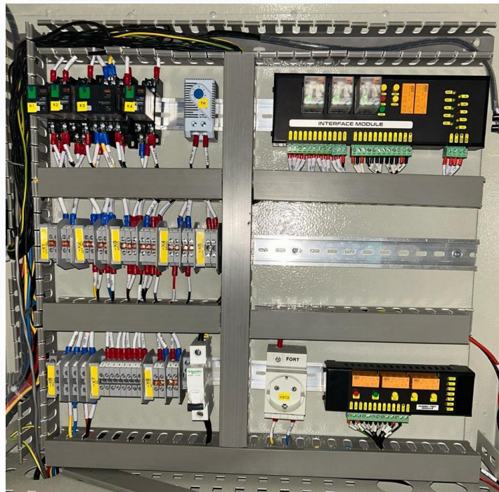
Gambar 3.9 Hasil perakitan komponen interface , dummy , relay .
