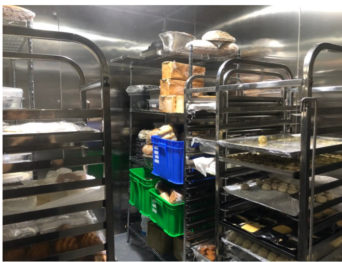
(Source: marriott.com) Figure 2.18 Walk in Freezer
