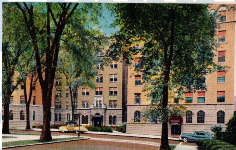
Gambar 2. 1 Gedung Sheraton Hotel Massachusetts
