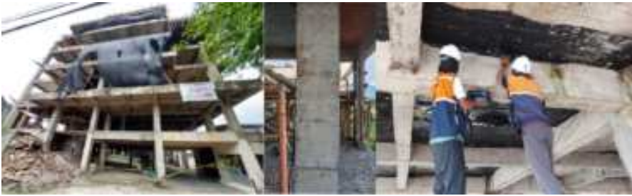
Fig. 1. Documentation of construction defects (left), horizontal assessment sample on slabs and documentation of structural assessment for beams and columns (middle and right).
