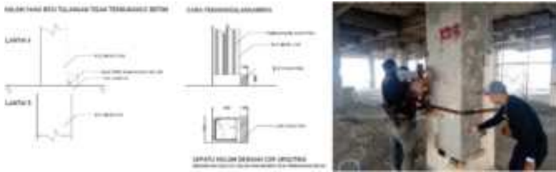
Fig. 6. Retrofit Strategies of Construction Defect of Mid-Rise Building using UHPC for columns shoes and CFRP for wrapping columns.
