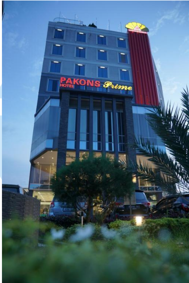
Gambar 2.1 Gedung Pakons Prime Hotel Tangerang
