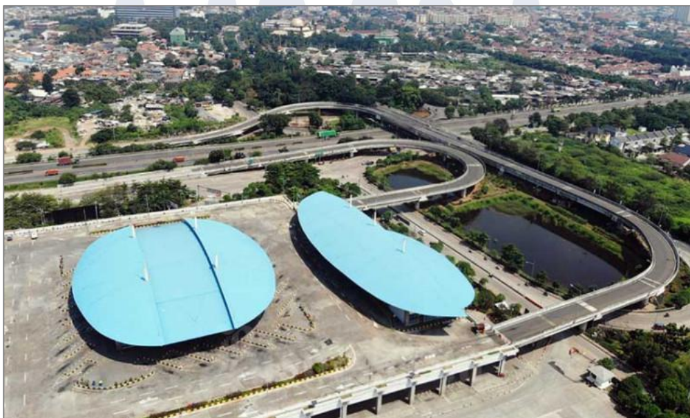
Gambar 2.17 Terminal Terpadu Pulo Gebang Sumber: Himawan L Nugraha (2020)
