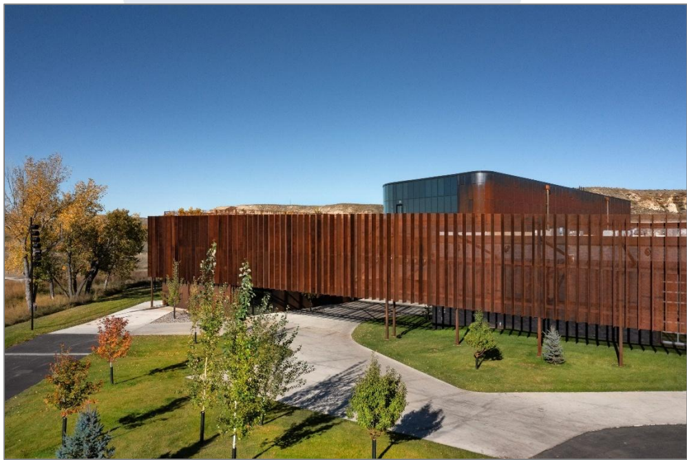
Gambar 2.9 EMIT HQ Sumber: CLB Architects (2023)
