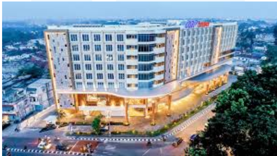
Gambar 2. 1 Gedung Hotel BW Luxury Jambi
