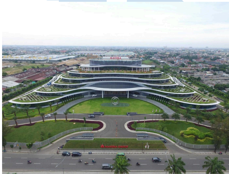
Gambar 1.1 Gedung Head Office Mayora
